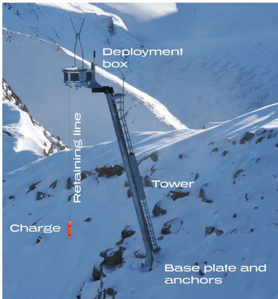
Figure 1 – Wyssen Tower with Deployment Box
