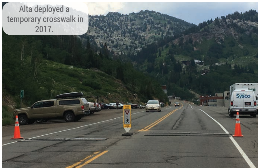
UDOT and Alta staff implementing a temporary center median.
